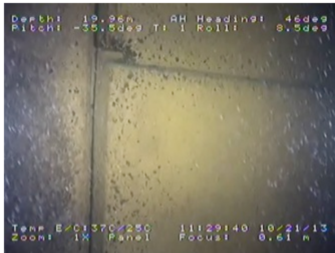
Upstream dam face inspection
