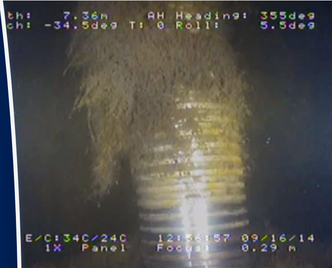
Verifying Valve operations
